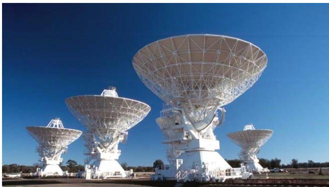
Visitors are welcome to drop in to the CSIRO's Australia Telescope complex where astronomers, with the aid of the Compact Array - a series of six 22-metre diameter antennas, are listening in to everything that's happening in the depths of outer space. The gigantic skeletal structures that each weigh 270 tonnes and move along a three kilometre long track, are an impressive sight, and tower over the
